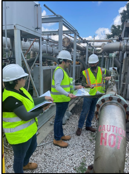
Flare system sampling in a South Florida landfill – Hydrocarbon Gas / Fuel Gas service testing
